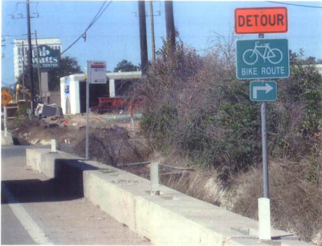
Example of detour sign placed on a bike route sign.
